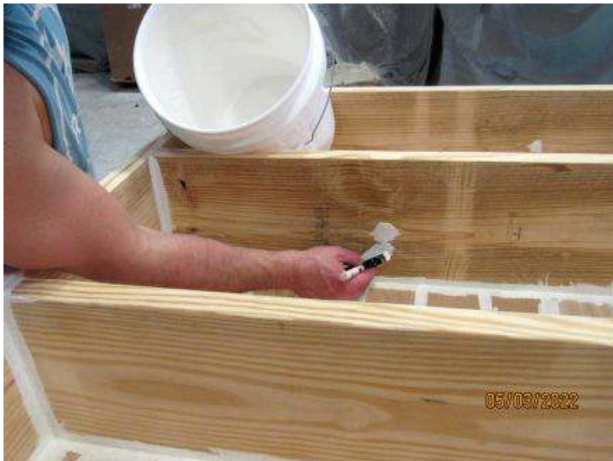
Photo No. 4 Applying coating to joints
