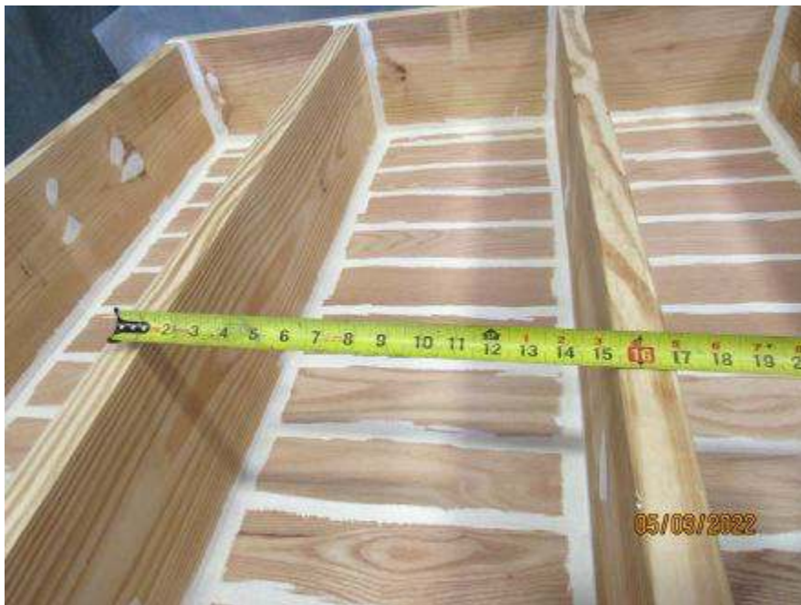
Photo No. 6 Joist spacing
