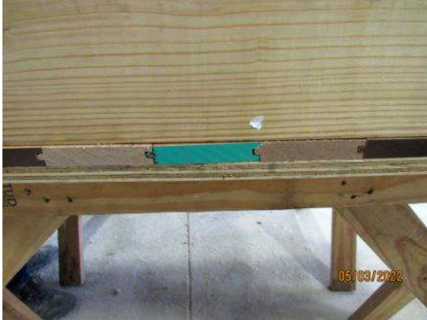
Photo No. 3 Red oak subfloor
